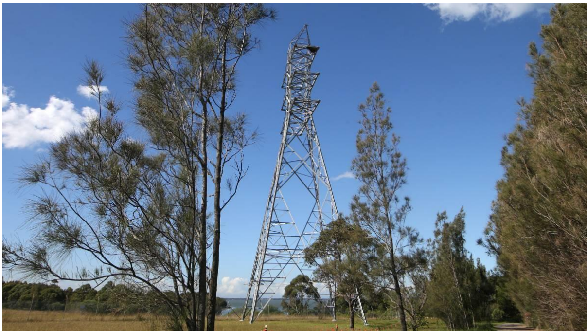
This tower is the only steel grid transmission tower that will be preserved, as a family of ospreys have made their nest at the top. Picture by Sylvia Liber
