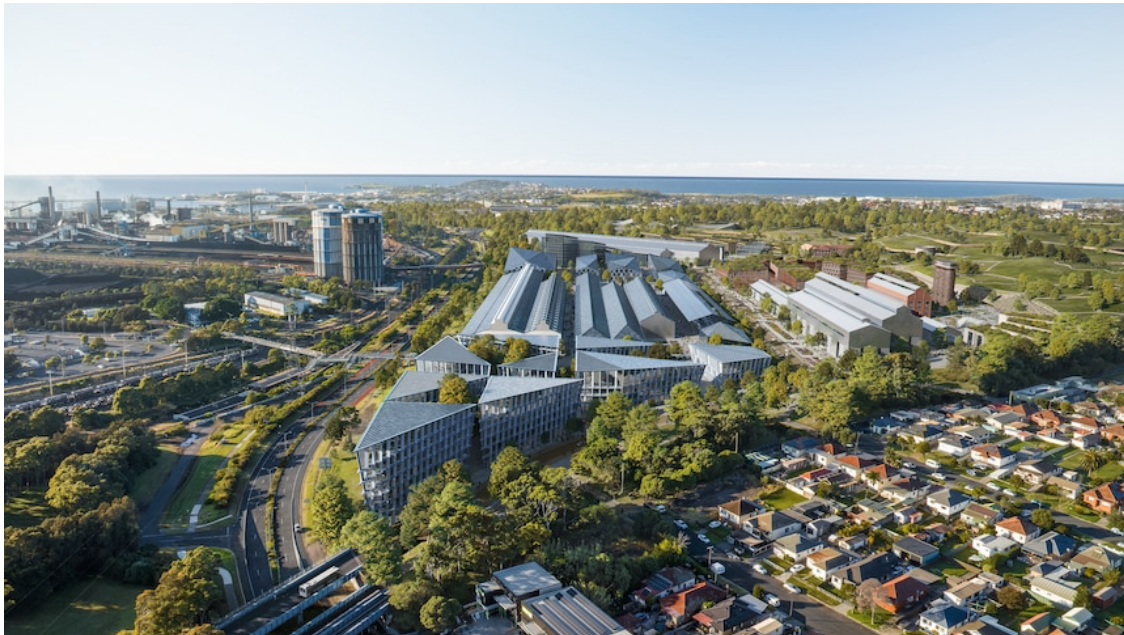
BlueScope Steel will redevelop 200 hectares of industrial land surplus to requirements. (Supplied: BlueScope Steel)
